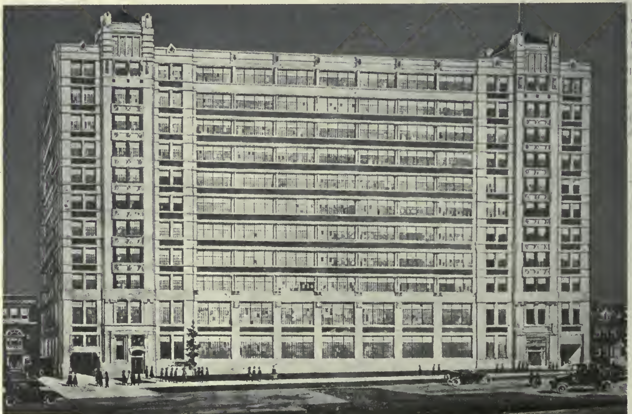
Fig. 1—The Robt. Simpson Co.'s. New Mail Order Building on Mutual Street, now under construction.
